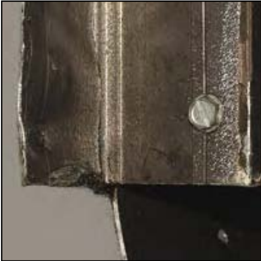
Mitered corner screwed together
