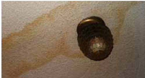
Allow water to drip from light fixtures, but remove the glass bowl to empty trapped water.
