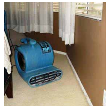
Air circulating fan for removal of moisture.
