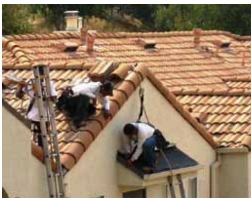
Sectional roof replacement
