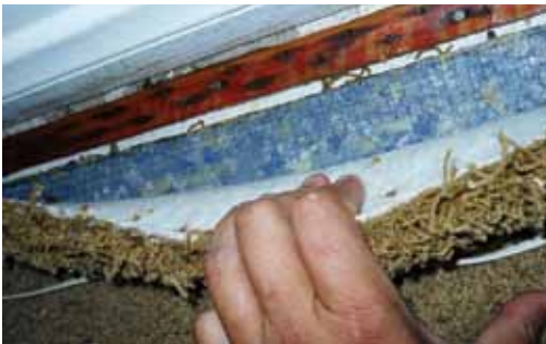
Lift wet carpeting and place towels at floorboards.
