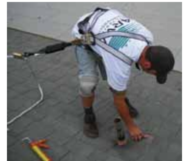
Temporary repairs - above and left
