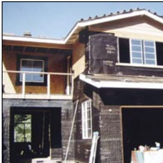
Paper behind stucco
