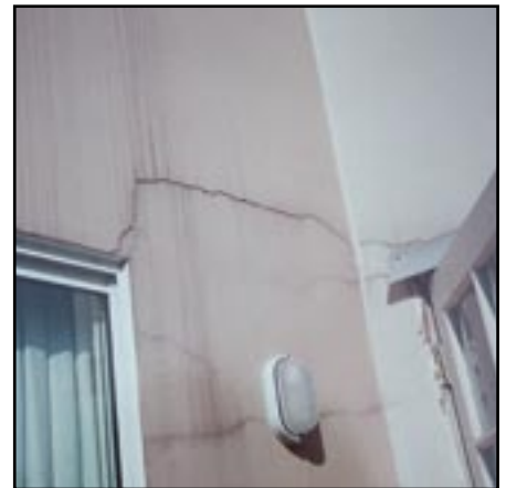
Stucco cracking
